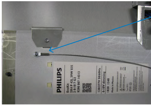
Picture D. Cable attached
