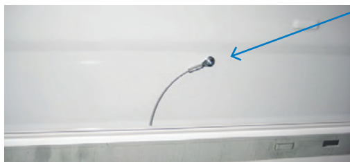
Picture H. Cable attached with self-drilling screw
