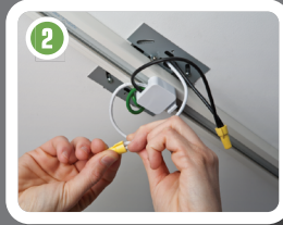
2 Connect track to mounting plate and wire.
