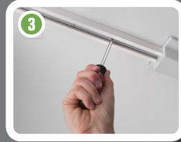
3 Attach track to ceiling.
